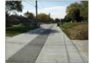
B. Permeable Concrete Alley
