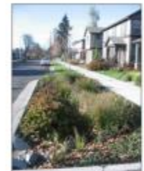
D. Sidewalk Retention Planter
