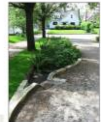
E. Curb Extension Retention
